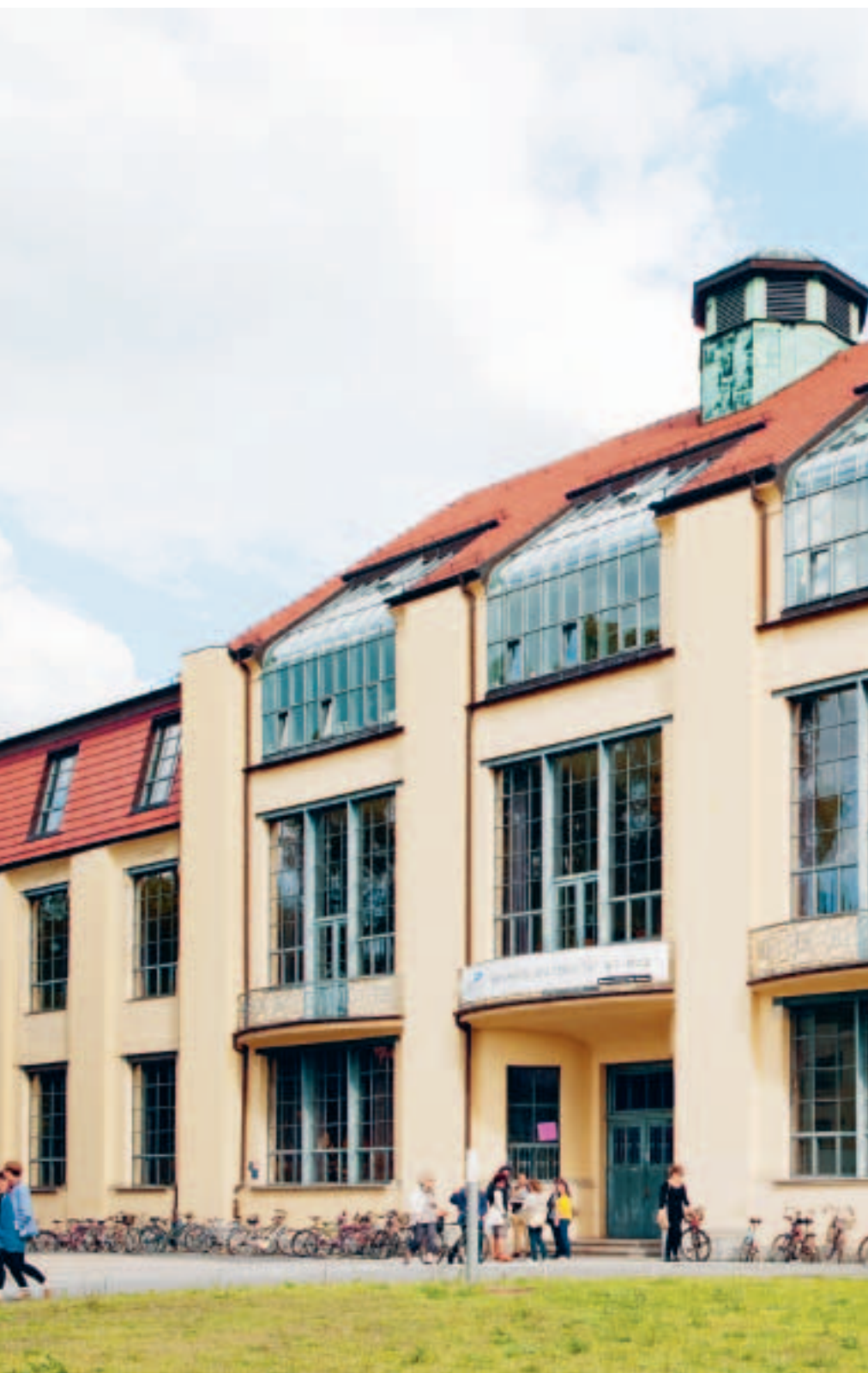
Bauhaus University, Main Building
